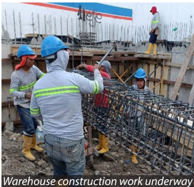
Warehouse construction work underway
